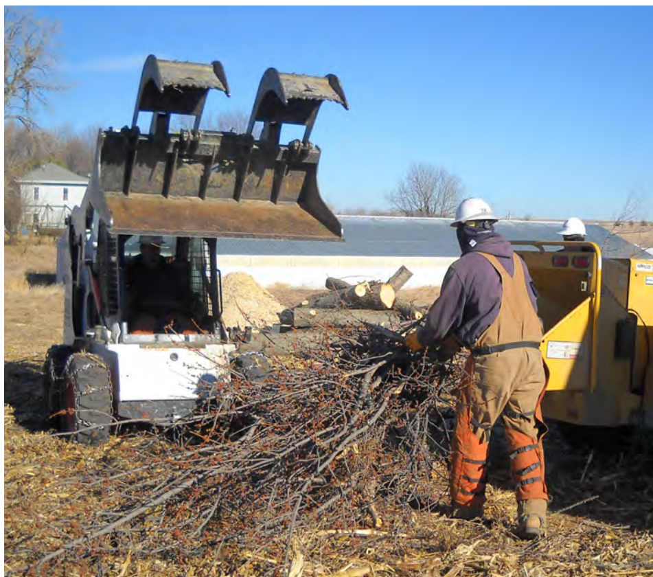
Crew foreman Tom Berkenpas feeds brush into a wood chipper in rural Cherokee County. The snow-free winter has been perfect weather for tree-trimming, an essential part of maintaining NIPCO’s system reliability. Overgrown trees are a hazard to overhead electric transmission and distribution lines. ❖ (Photo by Roger Armstrong)
