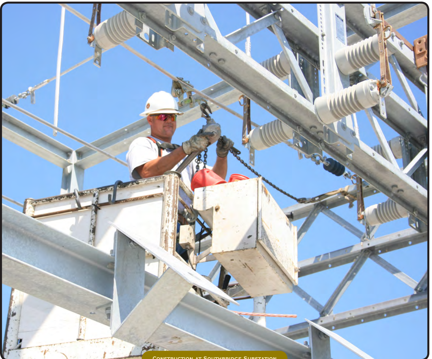
CONSTRUCTION AT SOUTHBRIDGE SUBSTATION
