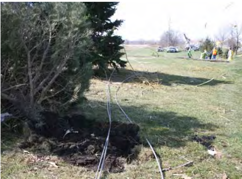
Broken conductor from NIPCO's tie line lies on the ground south of the Mapleton municipal substation while NIPCO crew members in the background remove the stump of a broken pole.
